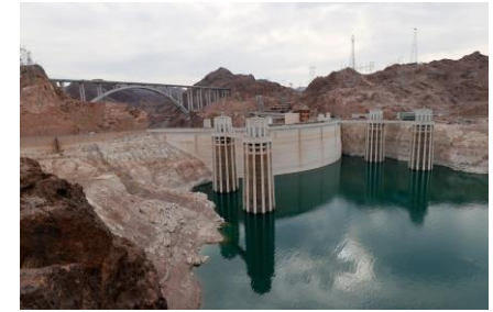
Hoover Dam is a concrete arch-gravity dam in the Black Canyon of the Colorado River, on the border between the U.S. states of Nevada and Arizona
